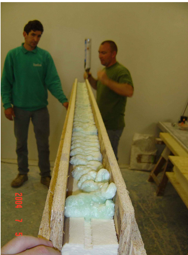
Photo 3 Applying the urethane expanding foam
